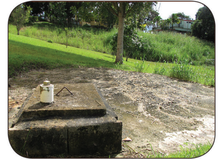
Keep septic tanks sealed.
